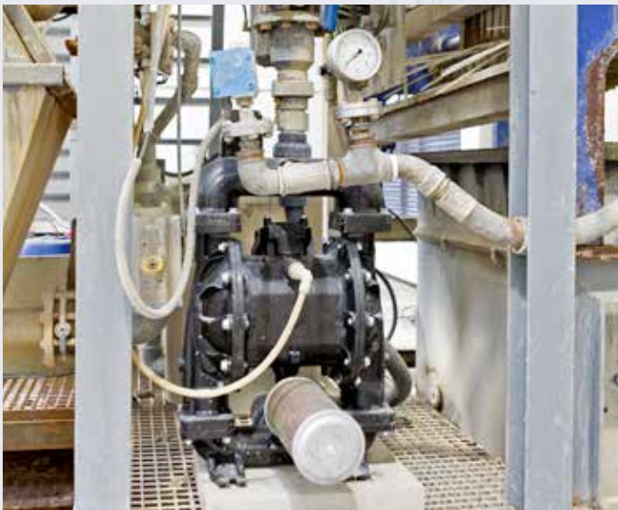
High suction lift reduces pump delivery.
